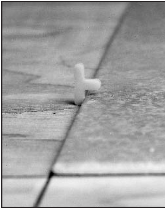
Fig. 13 - Use spacers with one leg removed.
