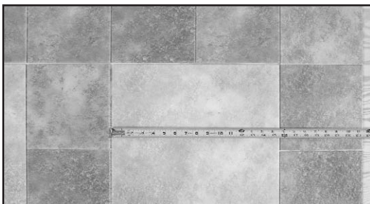
Fig. 23- Determine the dimensions for the pattern repeat.
