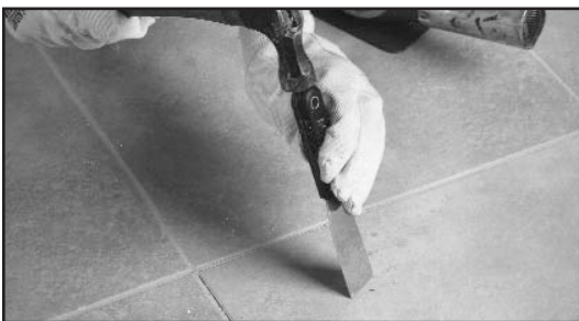
Fig. 38 - Drive a putty knife into the heated area and pry upward.
