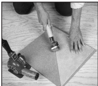
Fig. 28 - Roll the cut edge to form a slight radius.
