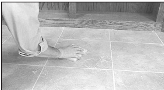
Fig. 31 - Use a 3M white, nylon pad to loosen grout residue.
