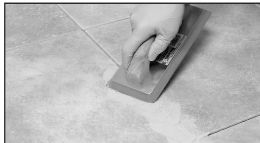
Fig. 29 - Pack the grout into the joints.
