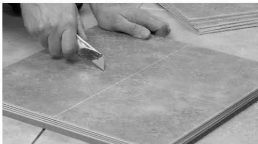
Fig. 4 - Score with a sharp utility knife.
