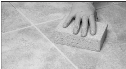
Fig. 32 - Wipe diagonally across the joints to remove excess water.
