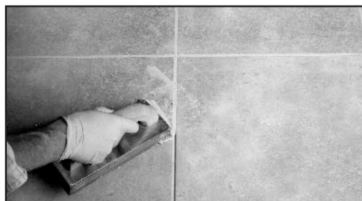
Fig. 30 - Extend grout a few inches into the next row.
