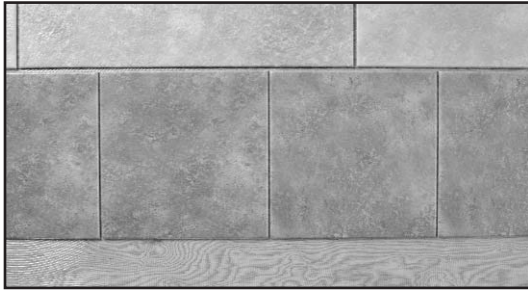
Fig. 22- An alternative to using different spacer sizes is to off-set the joints.
