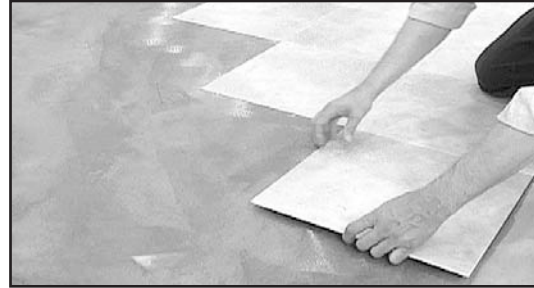
Fig. 16 - Install ungrouted floors following a stair-step pattern.
