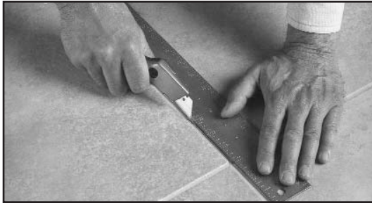
Fig. 37 - Cut along the center of the grout line after heating it.
